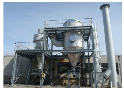
Fig.4: explosion proof exhaust filtering unit
